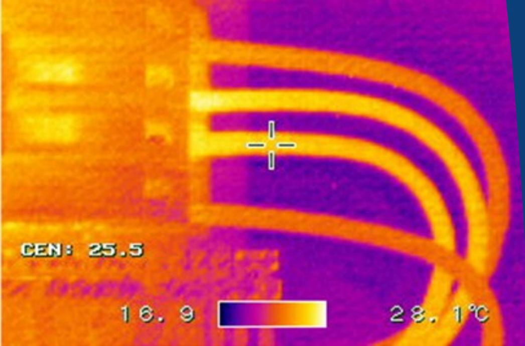
the engineer to a potential problem. The engineer will be trained to recognise whether the heat is sufficient to warrant further investigation, upon which the client will be notified. Generally speaking, thermal images can be taken by simply removing the cover or barrier to a piece of electrical distribution equipment, and does not require isolation.
